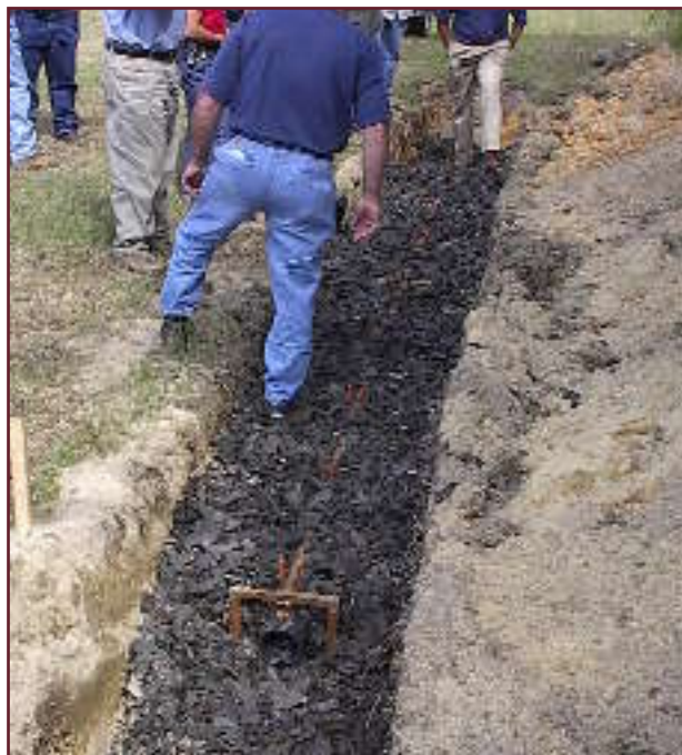
This demonstration installation of tire chips in a septic system in North Carolina featured the use of a steel brace for supporting the distribution pipe while the chips were loaded into the trench. Photo courtesy of Tim Warren.
